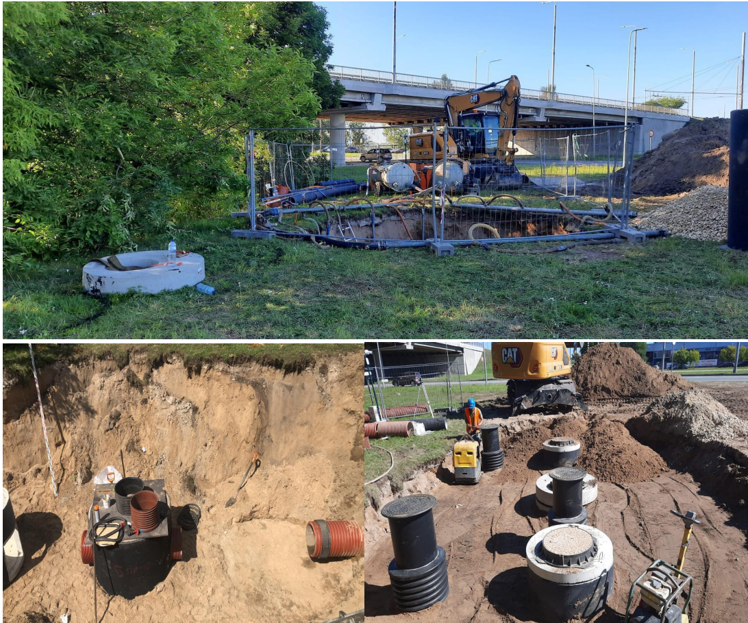
Construction site where the vertical hydrodynamic separator is installed
