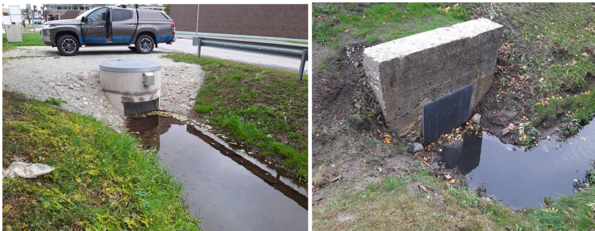
Constructed trash screens in demo sites 2 (Left) and 3 (Right)
