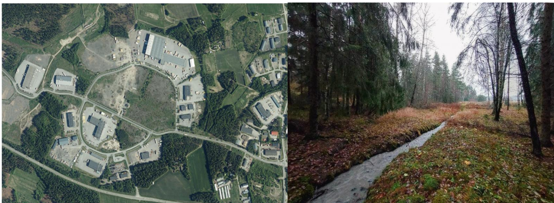
Catchment area of the Lieto pilot consists of an industrial area (left). Location of the stormwater treatment solution prior to building (right).
