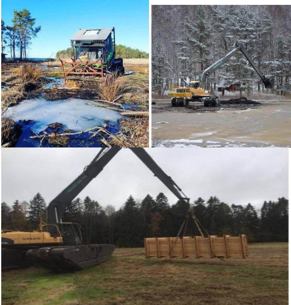
Cleaning and material transport in the area for constructing the wetland
