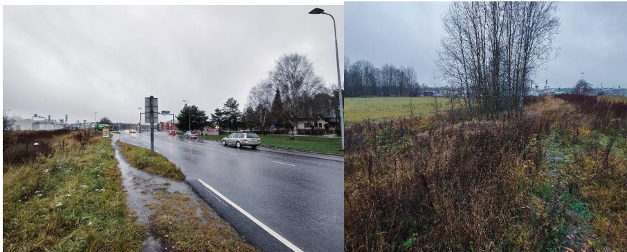
Catchment area of the Turku pilot consists of a road area (left). Location of the stormwater treatment solution prior to building (right).
